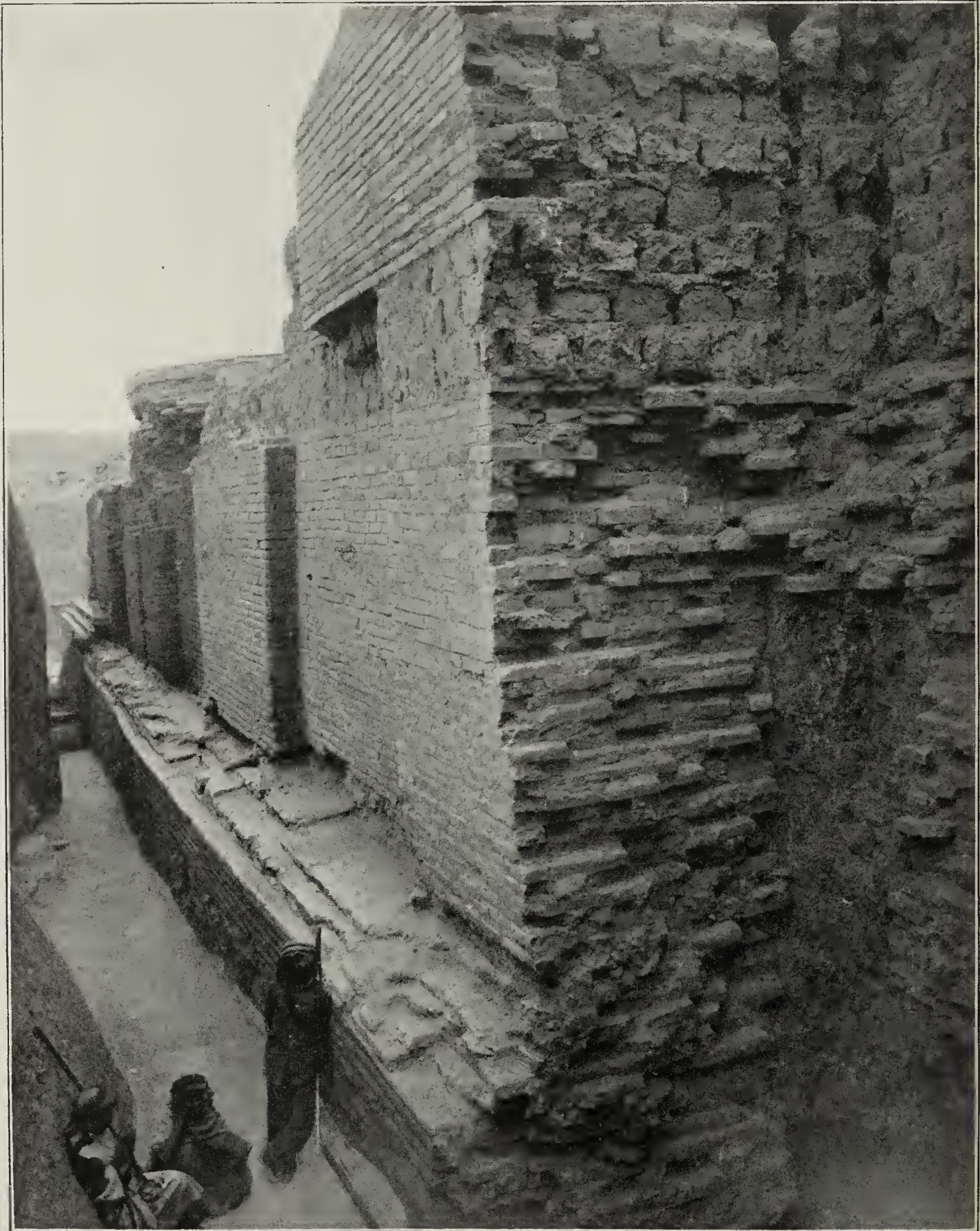
PANELED FACE OF ASSUR-BANI-PAL'S ZIGGURAT [FIG. 7]
